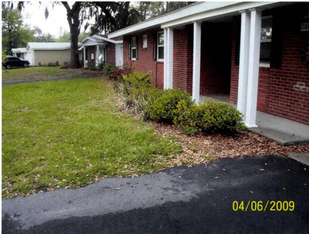
Picture 1: UST 268Beech excavation site. Tank was located beneath the two closest shrubs.
